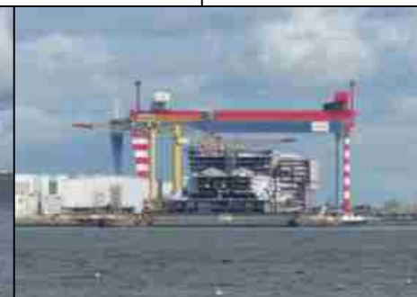
A cruise ship under construction
